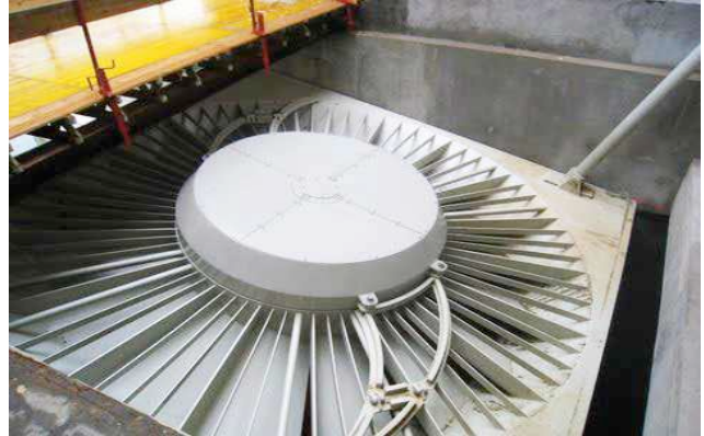
Fig. 7. Early testing of the VLH MJ2 turbine indicates the design is promising for eel passage.
