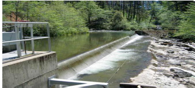
Fig. 3. The Montgomery Creek intake in California is an example of a Coanda screen, a curved or planar inclined screen with tilted wires designed to shear off bottom flow. The geometry allows efficient diversion of clean water with fine mesh filtration so that fish and debris pass over while clean water falls through.
