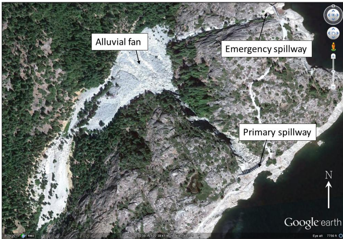
Figure 21: Aerial view of spillway showing alluvial fan of eroded material (note the walkway across the primary spillway is approximately 300 ft long for scale).
