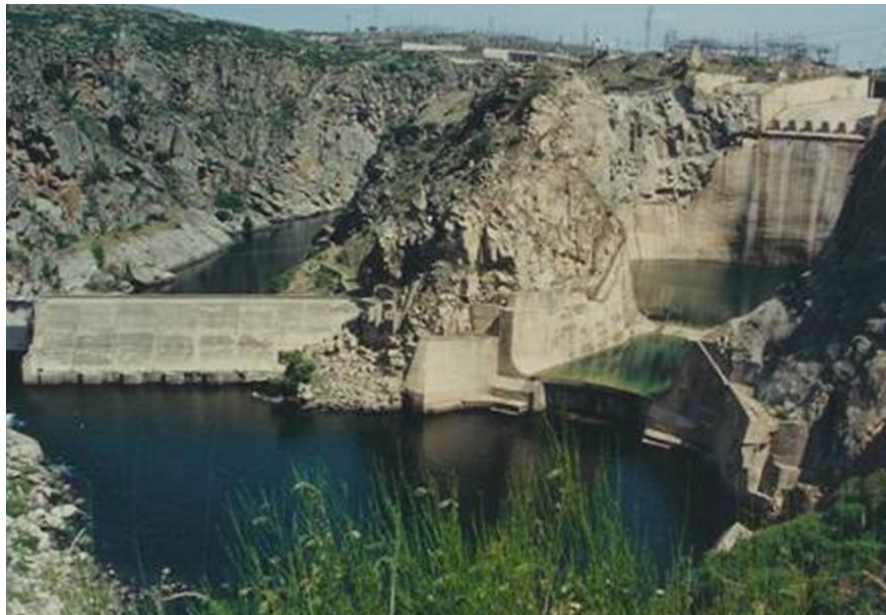
Figure 2: Scour remediation at Ricobayo (note extensive excavation and concrete work in addition to flow splitters on the spillway lip to dissipate hydraulic energy).
