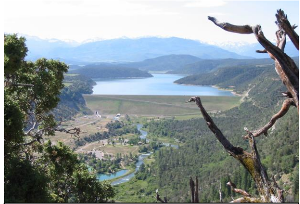
The 8 MW hydro project at Ridgway Dam in Colorado, completed in June 2014, was made possible by $15M in 2% loan funding provided by the Colorado Water Resources and Power Development Authority and the Colorado Water Conservation Board.
